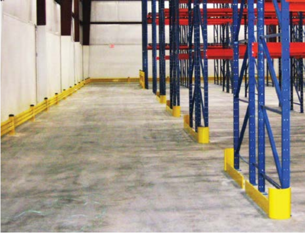
Perimeter protection and rack guard
