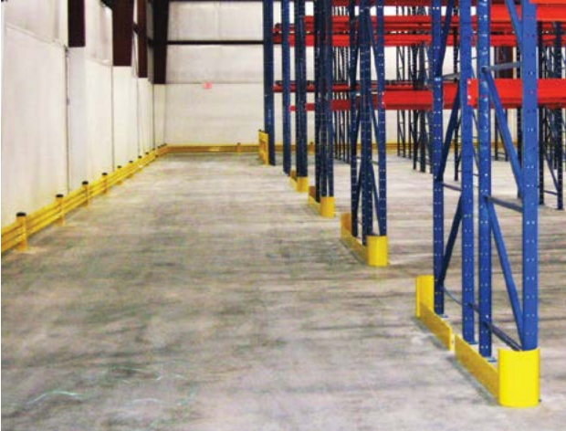
Perimeter protection and rack guard
